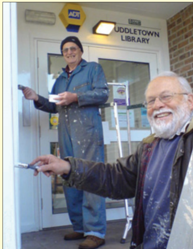
Mick Oddy (left) and Bill Maunder re-painted the shabby library lobby over the Easter bank holiday. A third FoPL member (who wants to remain anonymous) has offered to pay for the paint.
